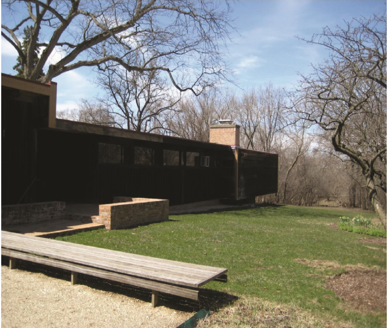
Schweikher House, 645 Meacham Road Schaumburg, IL 60193
