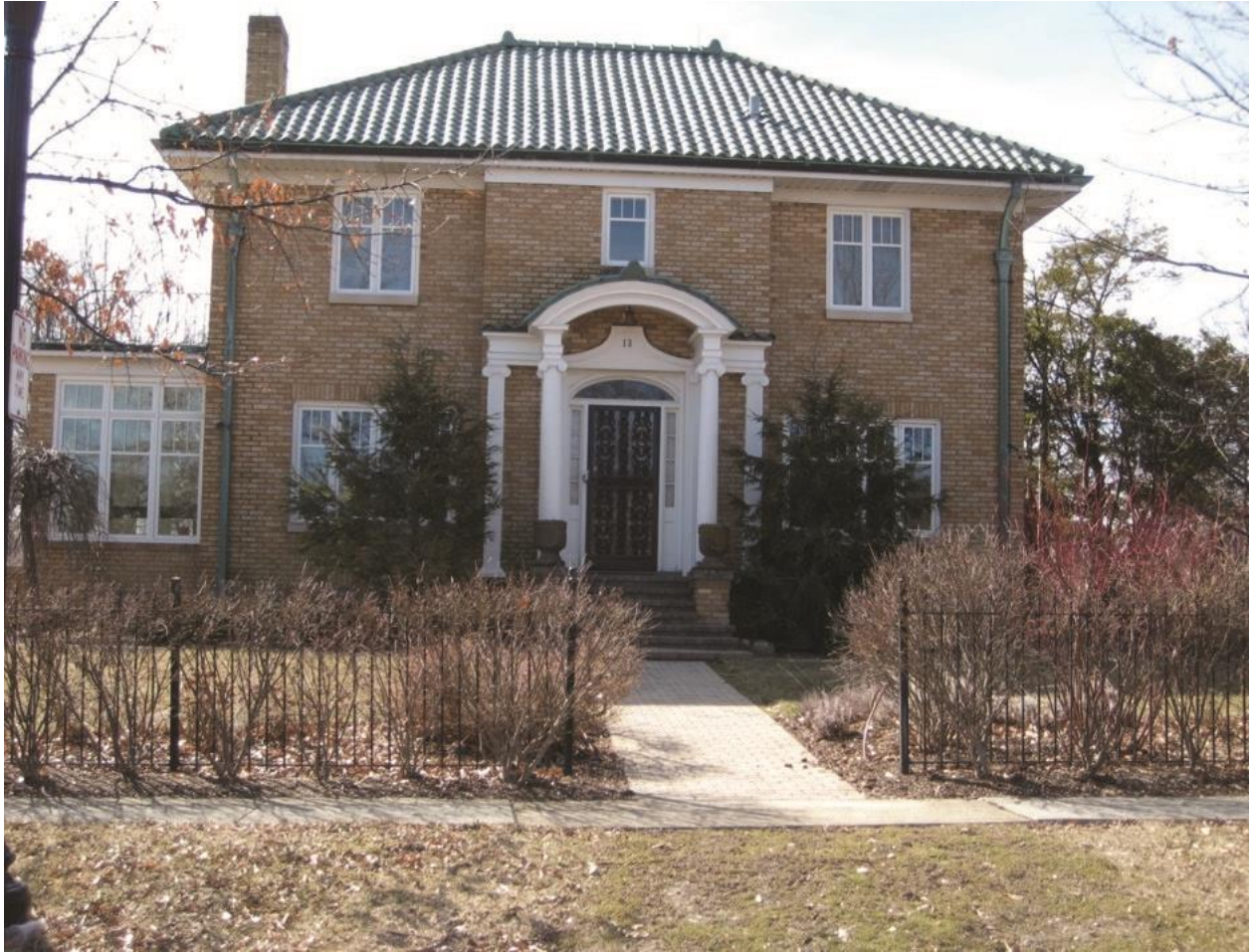
Frank Lengl House, 13 Quindel Avenue Schaumburg, IL 60193
